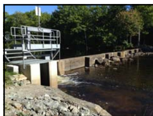
Fig. 1: Pushaw Lake outlet dam in summer— fishway on left. (Gate is closed) Photo credit: Rich Dressler
