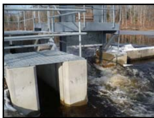
Fig. 2: Pushaw Lake outlet dam in early winter with gate open (fishway on left) Photo credit: Rich Dressler
